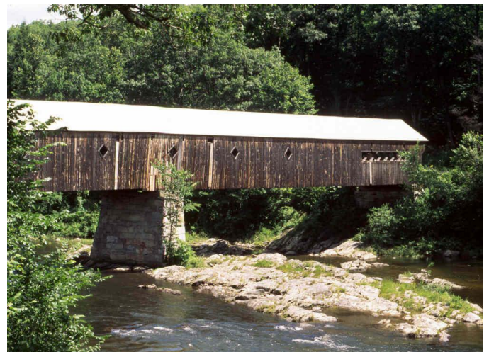
West Dummerston Bridge, Photo by Joe Nelson, July 1995
