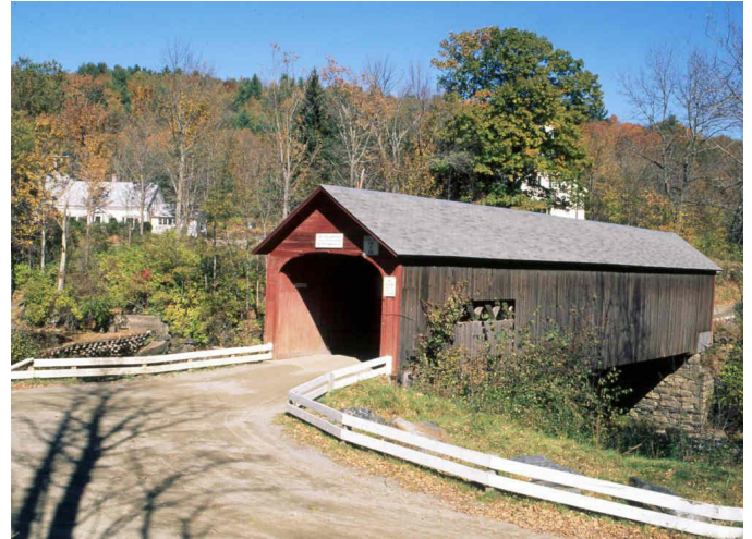
Green River Bridge, Photo by Joe Nelson, September 1995
