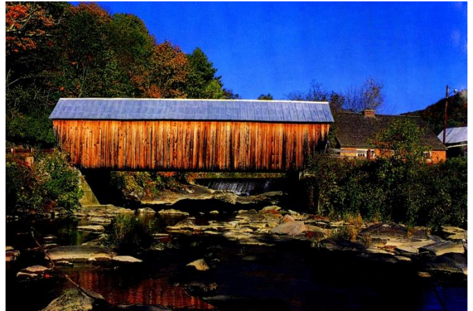
Mill Bridge, photo by Joe Nelson, 1997
