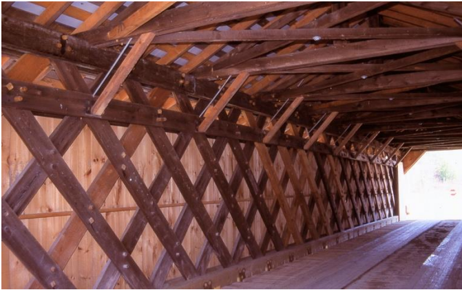
Hopkins Bridge, by Joe Nelson, June 1, 2000
