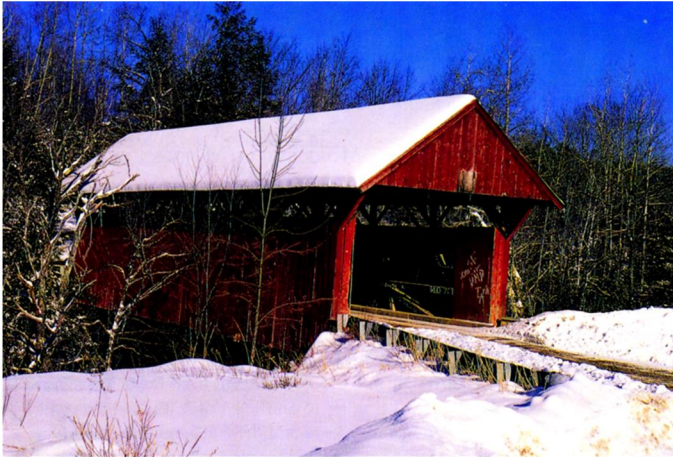
Red Bridge, photo by Joe Nelson, 1997
