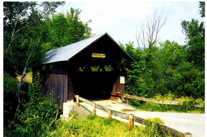
Gold Brook Bridge, photo by Joe Nelson, 1997
