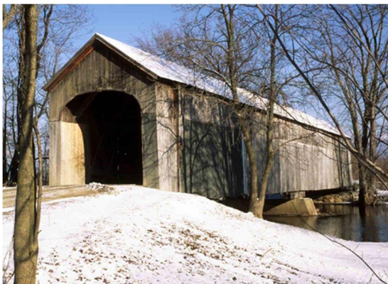
Salisbury Station Bridge by Joe Nelson
