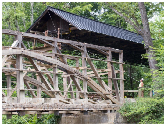
Seguin Bridge During Repair Work Photo Courtesy Melrose Huff
