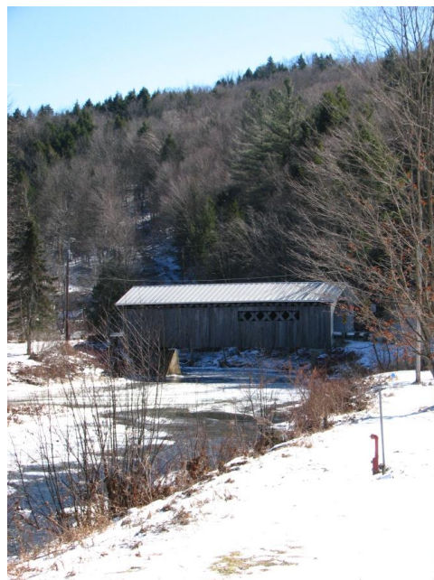
Comstock Bridge, Montgomery
