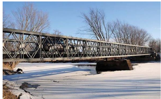
Photos courtesy Addison County Independent & Trent Campbell
