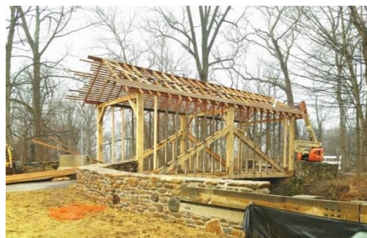
Roddy Road Bridge, Frederick County, Maryland Michael Rudnick Photo, January 17, 2017
