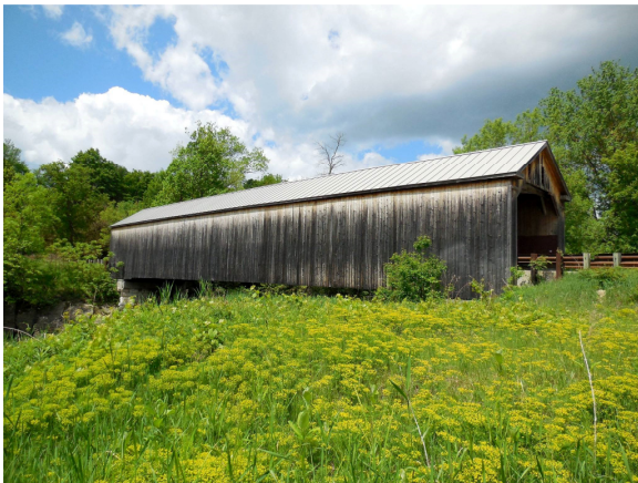
Sanderson or Upper Bridge (45-11-02 #2) May 22, 2015.
