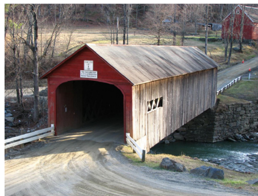
Green River Bridge, Guilford, VT Bill Caswell Photo, April 21, 2014]
