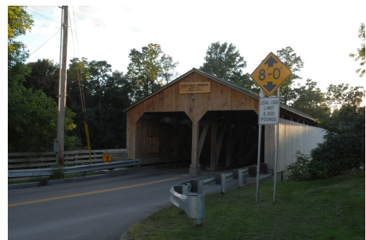
Pulp Mill Bridge, Middlebury/Weybridge
