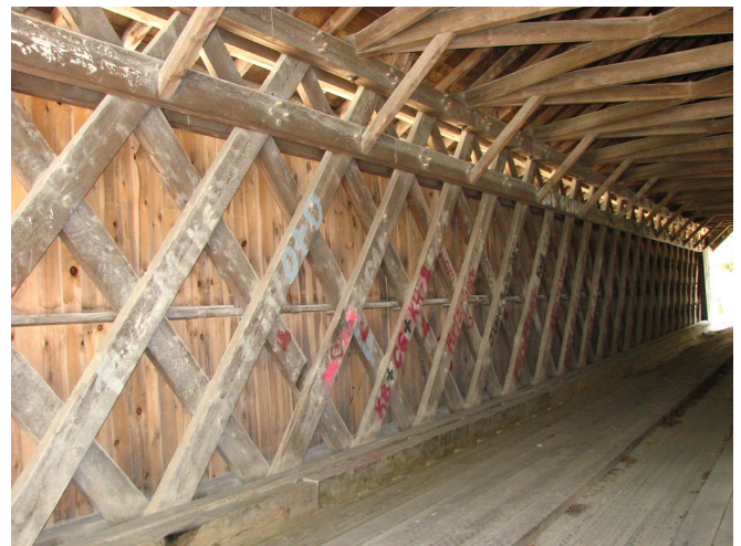
Interior of Brown Bridge, Shrewsbury, Vermont
