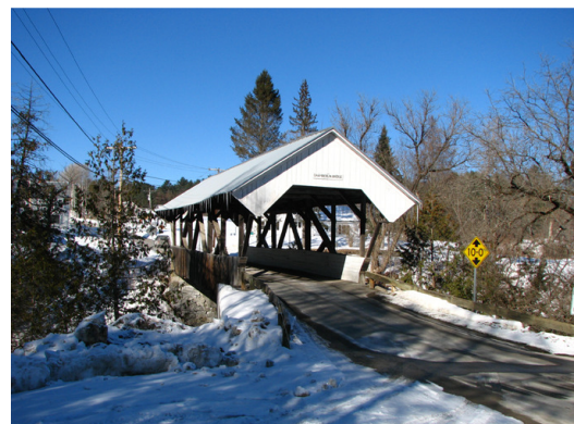
Chamberlain Bridge, Lyndon, VT, March 3, 2014
