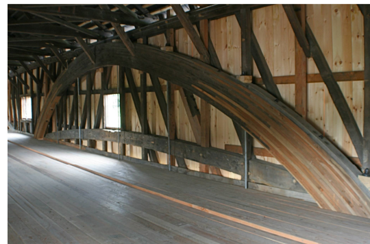
Interior of Bath Bridge, Bath, NH Scott Wagner Photo, August 16, 2014
