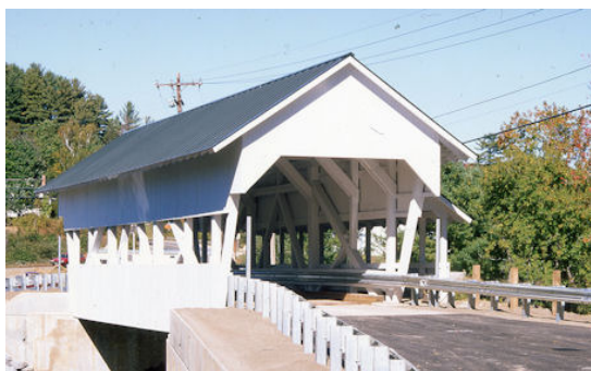
Millers Run Bridge, Lyndonville Photo by Joe Nelson 1995
