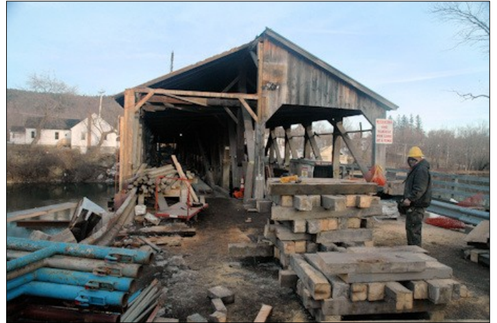
Pulpmill Covered Bridge Renovation Begun Photo by Ed Barna, February 27, 2012]
