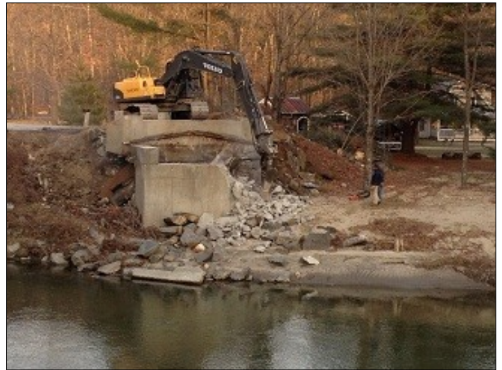
North abutment – December 14, 2011 by Adrienne Hitchcock
