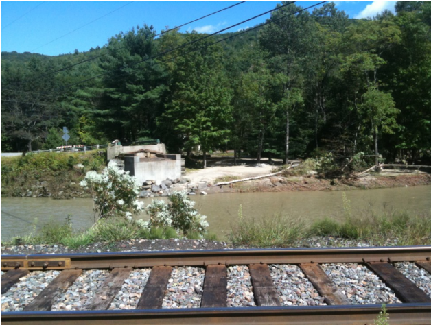
Bartonsville north abutment August 30, 2011 photo Ray Hitchcock
