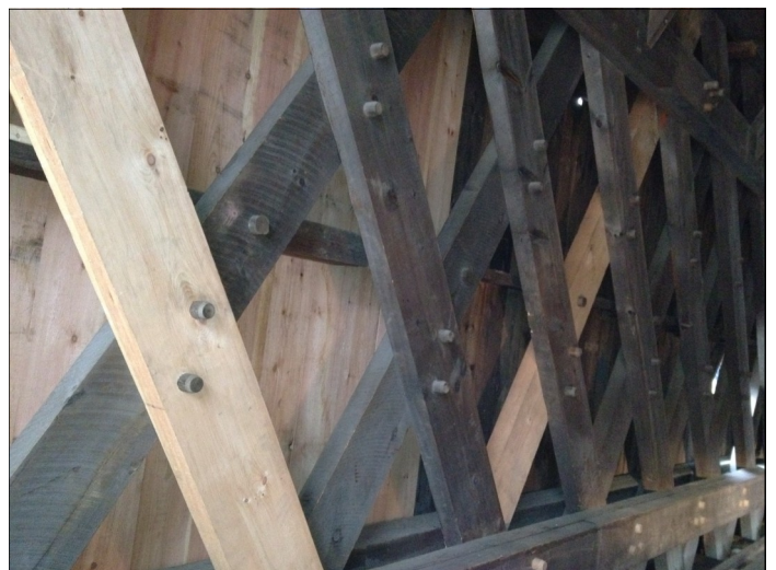
Hall lattice and siding repairs—Nov 29, 2011 photo by Ray H.
