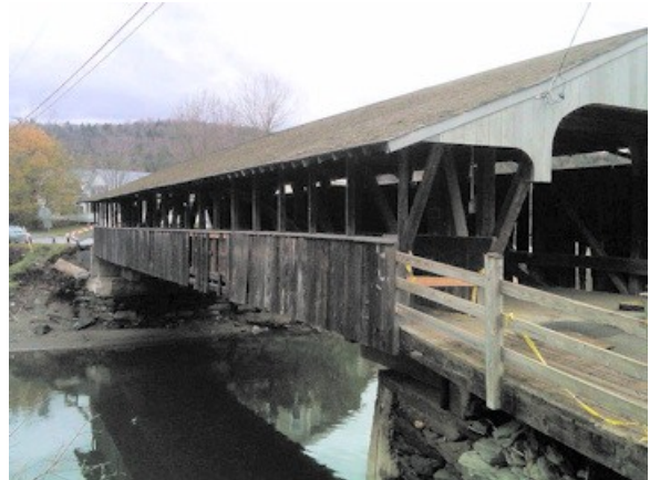
Waitsfield Bridge photo by Richard Hiscock 10/24/2011
