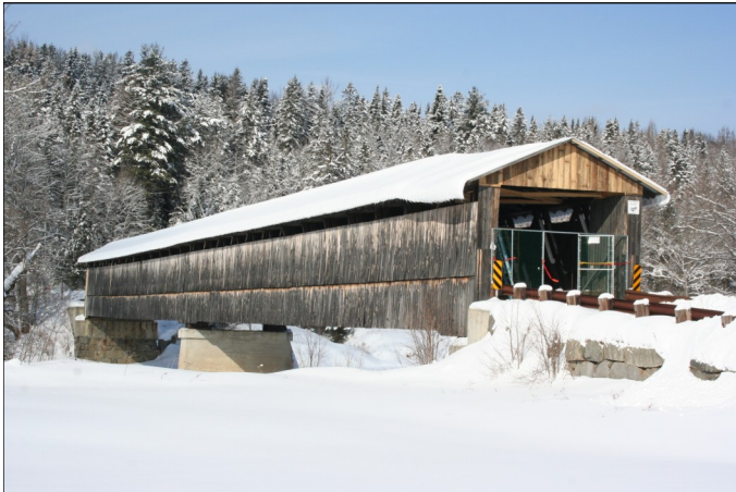
Mt. Orne Bridge closed for repairs – photo courtesy R. Durfee, Feb. 23, 2011
