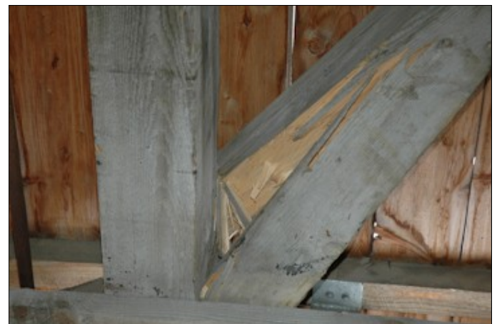
Cambridge Junction Bridge - Damaged Brace
