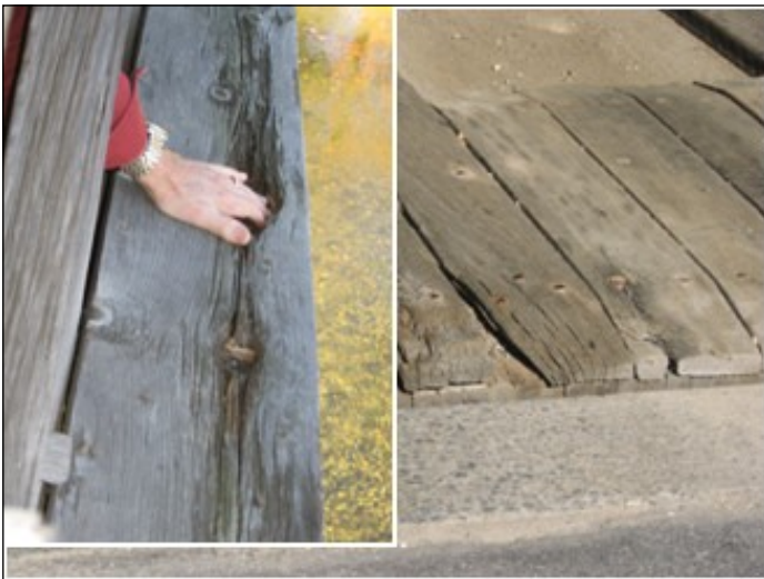
Damaged window sill Worn running plank Bartonsville Bridge—Photo by Ray Hitchcock Nov 2010
