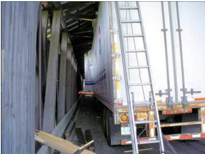
Truck wedged into Mount Orne Bridge, Photo from Pamela Maza Thurber, P.E. VTrans, June 6, 2006
