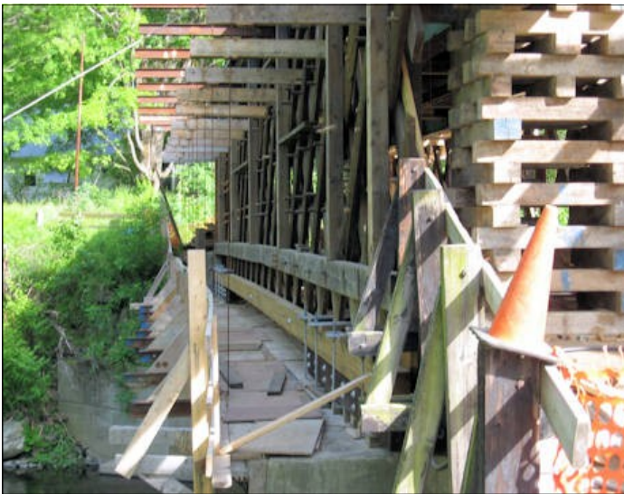
Upstream lower chord from west portal - Photo by Ray Hitchcock
