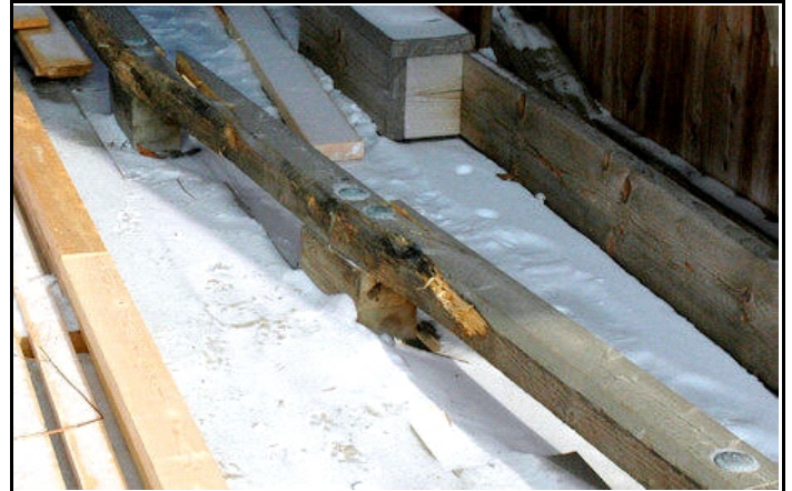
Cambridge Junction Bridge, Broken Curb-rail. Photo by Joe Nelson
