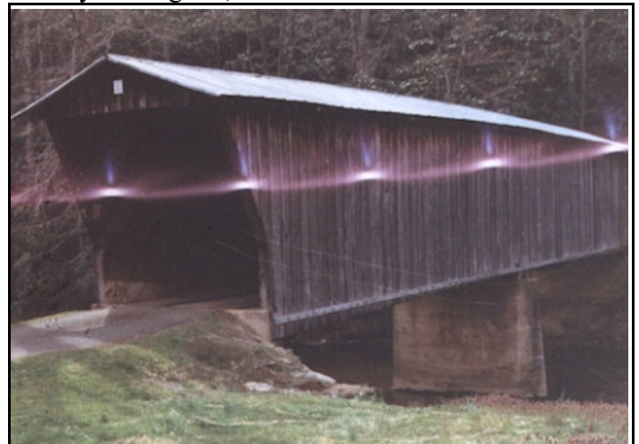
The Halos at the Bob White Bridge VA-68-01 Photo by Don Overman
