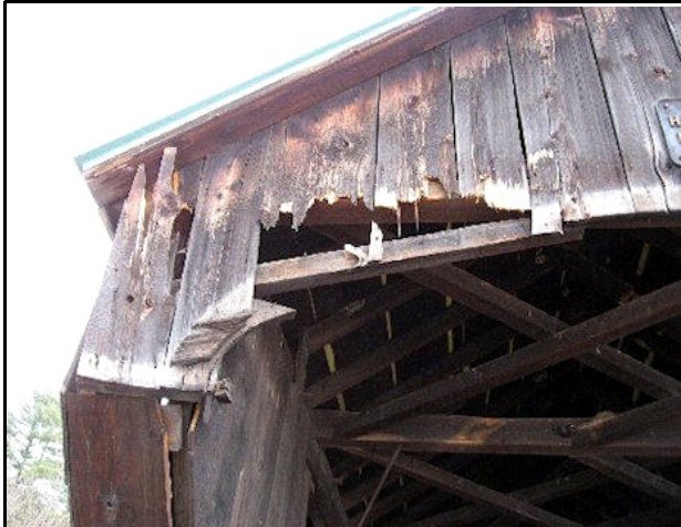
Worrall Bridge VT-13-10, Photo by Ray Hitchcock January 2009
