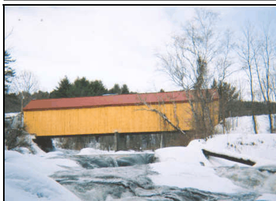
Union Village Bridge 45-09-05 Photo by Jack Teece, Feb. 2008
