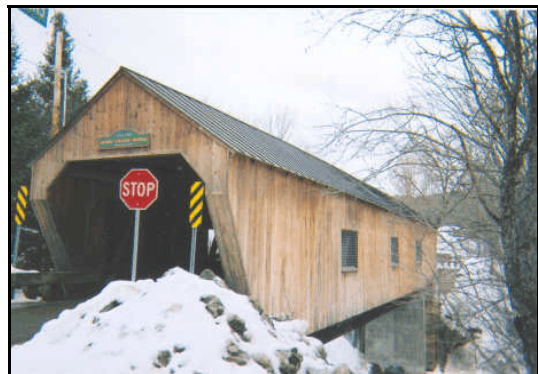
Sayers Bridge 45-09-06 Photo by Jack Teece, Feb. 2008
