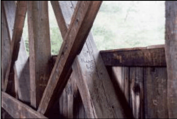
Truss at Sunday River Covered Bridge ME19-09-14, Photo By Trish Kane
