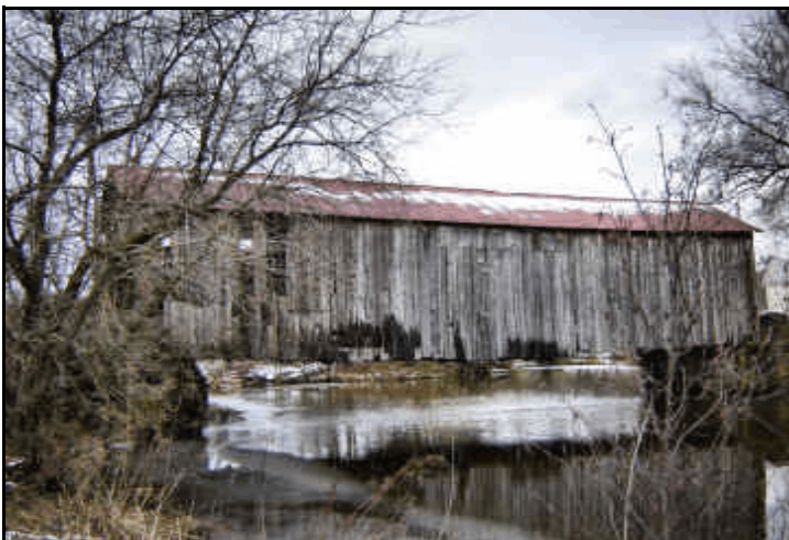
East Fairfield Bridge, WGN VT-06-03 Photo by Hoyle-Tanner & Associates, INC, 1/24/07
