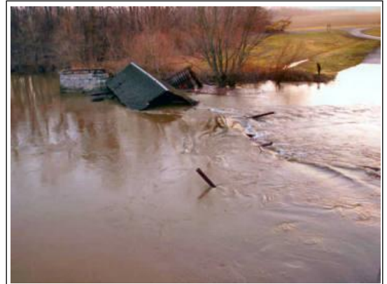
Bell Ford Bridge [WGN 14-36-03] January 4, 2006
