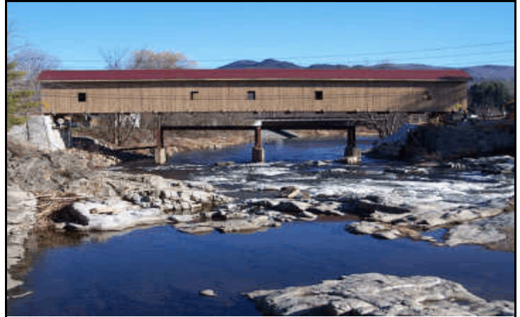
Side view of the Jay Bridge [WGN 32-16-01] sitting high over the abutments. Notice the new bridge behind the covered bridge and the old piers.
