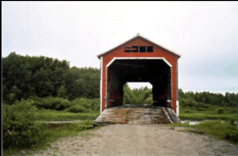
du Panache Bridge Photo by Gerald Arbour May 3, 2006
