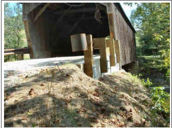
Slaughterhouse Bridge with new fire retardant coating Photo by John Weaver
