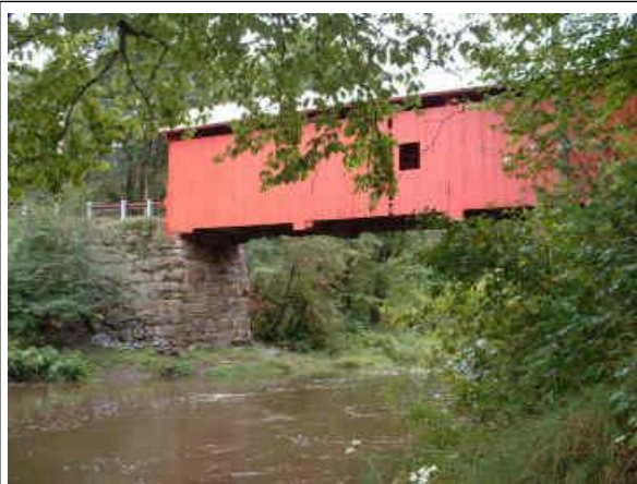
Moxley Bridge [WGN 45-09-01] approach work Photo by John Weaver
