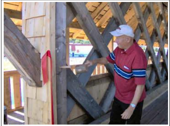
Dick Wilson drives in the last "trunnel" Sept 24, 2005
