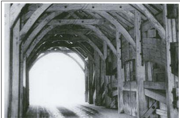
Horbenbrücke S-06-16. Photo by Konrad Meyer-Usteri
