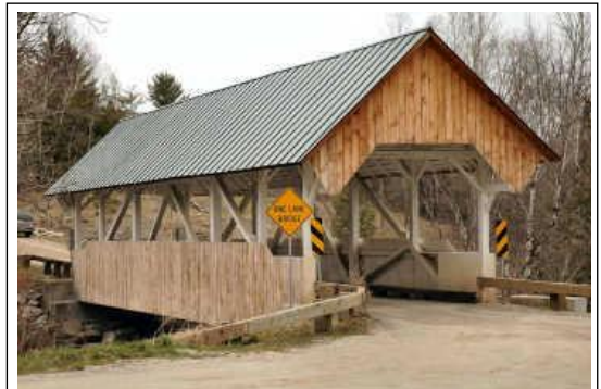
Greenbanks Hollow Bridge [45-03-01] in Danville. This bridge is a must-see. It has been recently renovated converting it from a cripple supported by piers and I-beams to a fully functioning, self supporting wooden covered bridge, just as it's original builder meant it to be. Photo by Joe Nelson
