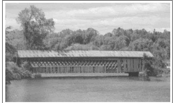
Pompanoosuc Village Bridge [45-14-67] Razed in 1954. From old postcard.
