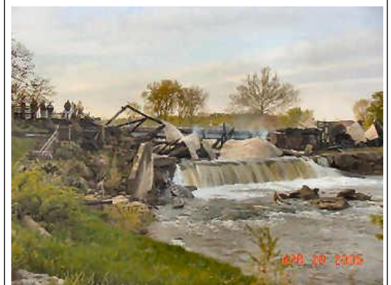
Bridgeton Covered Bridge fire. Photo by Cathy Harkrider May 28, 2005
