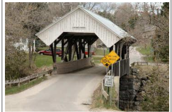
Chamberlin Bridge [45-03-04] located at York Street in Lyndon Corners, a short walk from the Grange Hall. Photo by Joe Nelson
