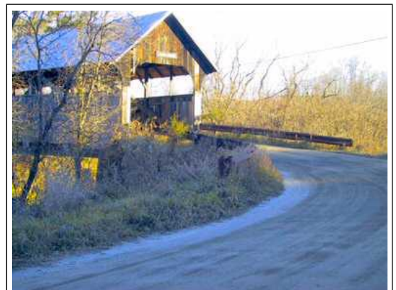
Coburn Bridge approach from the North
