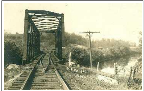
Fowler, Vermont railroad & covered bridge
