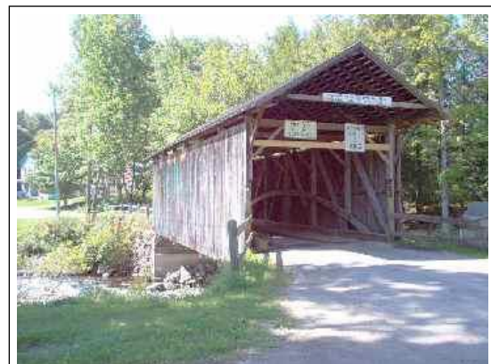
Salisbury Center Bridge NY-22-01 photo by Dick Wilson August 2004
