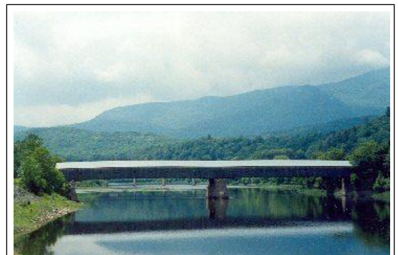
Windsor-Cornish Covered Bridge. Photo by Helga McGuire
