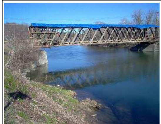
Buskirk Bridge [NY-42-02] Photo by Dick Wilson, April 16, 2004
