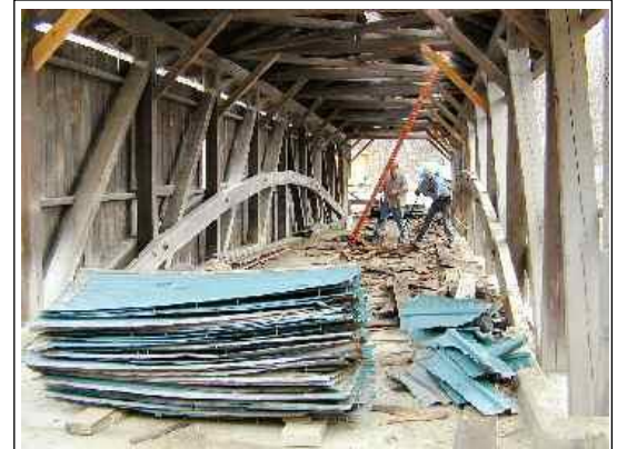
Removal of old metal roof reveals even older wooden shingles.
