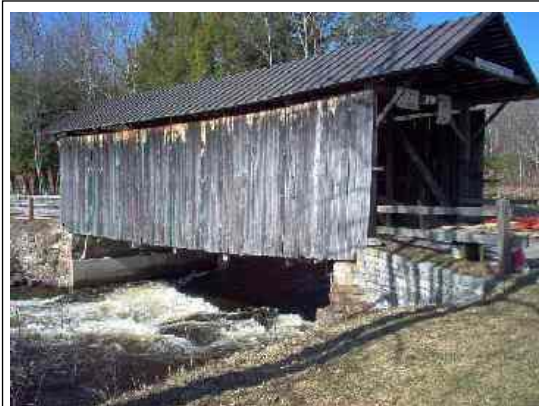
Salisbury Center Bridge [NY-22-01] Photo by Dick Wilson, April 16, 2004
