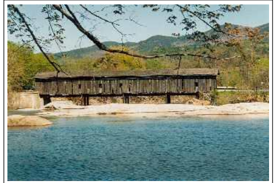
Jay Bridge (32-16-01) Photo by Dick Wilson May 1997
