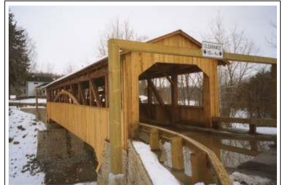
Knapps Bridge [WGN PA-08-01] Built in 1853 using the Burr Truss to cross Brown's Creek near Luthers Mills, PA. Renovated in 2002. Photo by Chuck and Nancy Knapp, March 21, 2003
