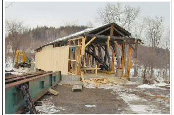
The siding is nearly complete on the downstream side.
