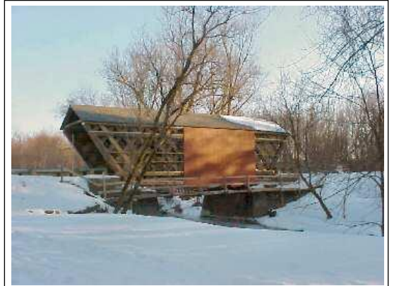
Cooley Bridge, downstream side
