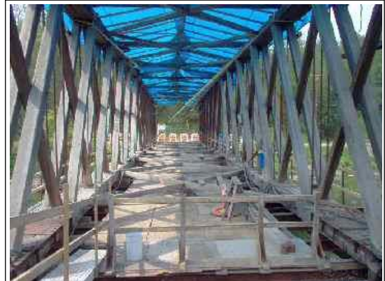
Buskirk Bridge [NY-42-02] Photo by Dick Wilson, July 5, 2004
