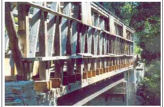
Union Village Bridge Photo by N. David Charkes September 2004
