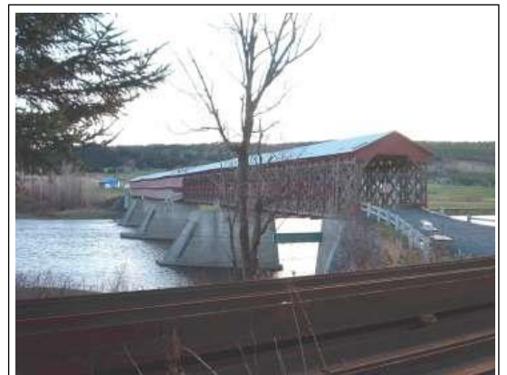
Perreault Bridge Repairs Underway Photo by Jimmy Veilleux, May 2003
