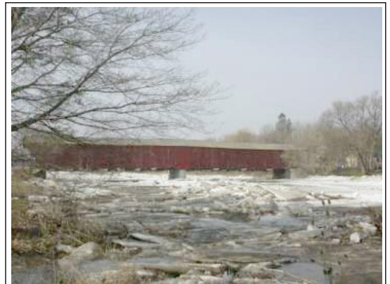
Kissing Bridge W. Montrose, Ontario, Canada Photo by B. Larrabee
