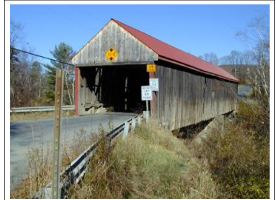
The truss used in the span is a unique adaptation of Herman Haupt's 1839 patent. The midstream pier was added in 1963. Photo by Joe Nelson, 1997.
