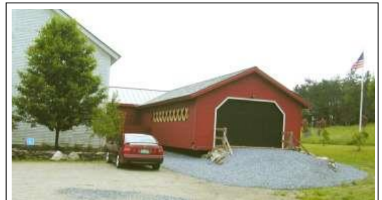
Vermont Covered Bridge wing at Bennington Center for the arts Photo by Joe Nelson, 6-14-03
