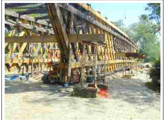
The multi-color timber shows the different species used in the new work; native spruce, southern yellow pine, and Douglas fir contrast with older timbers.
