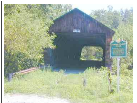
Hammond Bridge. "only a chain between two posts" Photo by Joe Nelson, Aug. 19, 2003
