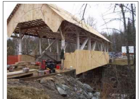
Greenbanks Hollow Bridge, Danville. Vt. (45-03- 01) Photo by Mert Leonard, 11-15-02
