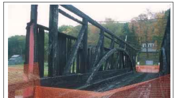
Ryot Bridge, Bedford County, Pa. (38-05-17) Photo by Joe Nelson, 10/16/02
