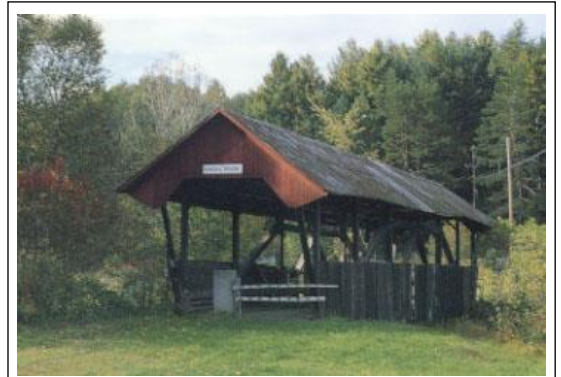
Randall Bridge at Lyndon, Vt (45-03-07) Photo by Joe Nelson, 1997
