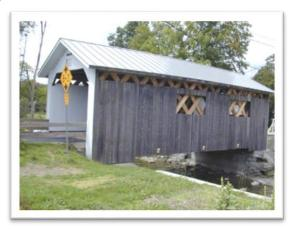
There is no salvage except for the roof, which was rebuilt after it was torn off in the winter of 1982 by a logging truck.
