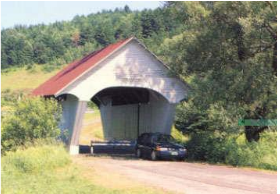
School House Bridge Photo by Joe Nelson, 1994
