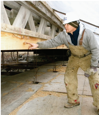
Project Superintendent Rich Butrimas points out one of the new oak pegs, or trunnels (also known as tree nails), used as fasteners. This is the traditional methodology of the covered bridge builder and used in securing the new section of the lowermost chord that has been grafted in.
