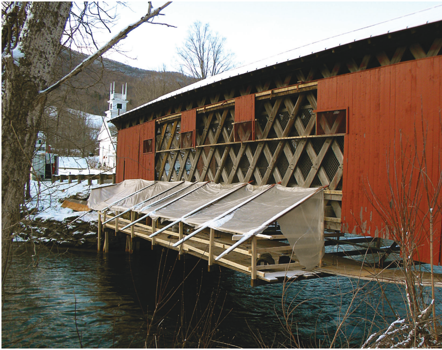
By January 30, parts of the bridge siding had been removed to gain access to the trusses and chords of the bridge. Plastic was used to cover scaffolding and provide protection from the weather as work progressed both under and on the upstream side of the bridge.
