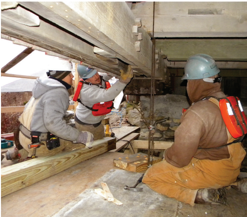
Project Superintendent Rich Butrimas points out one of the new oak pegs, or trunnels (also known as tree nails), used as fasteners. This is the traditional methodology of the covered bridge builder and used in securing the new section of the lowermost chord that has been grafted in.
