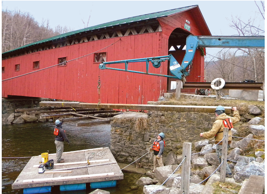
On January 25, 2012, the three-man crew from Wright Construction was hard at work, using a raft to serve as a temporary platform from which to hang scaffolding under the bridge. The damage inflicted by Tropical Storm Irene the previous August was apparent (below) in the outward bow in the downstream side of the bridge.
