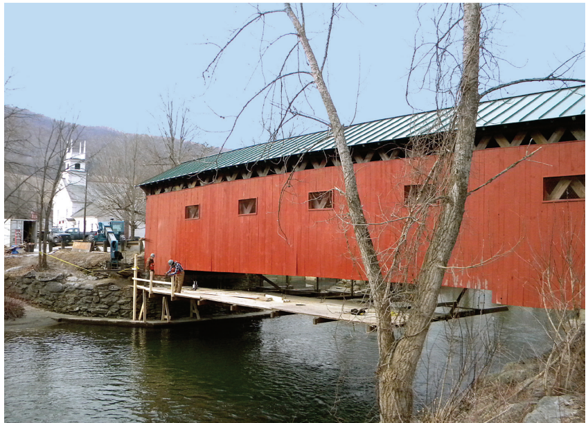
With new siding (that had been pre-painted in Wright Construction's shop) installed, the crew was busy taking down scaffolding when this photo was taken the day before the bridge opened to traffic.
