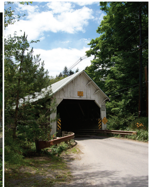
Williamsville's original bridge (above) served for more than one hundred years before being replaced, as Newfane selectman Gary Katz watched the final steps of the process.
