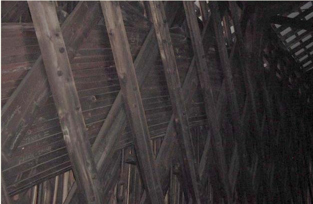
Wright's Bridge (Built 1906) – Newport, NH
