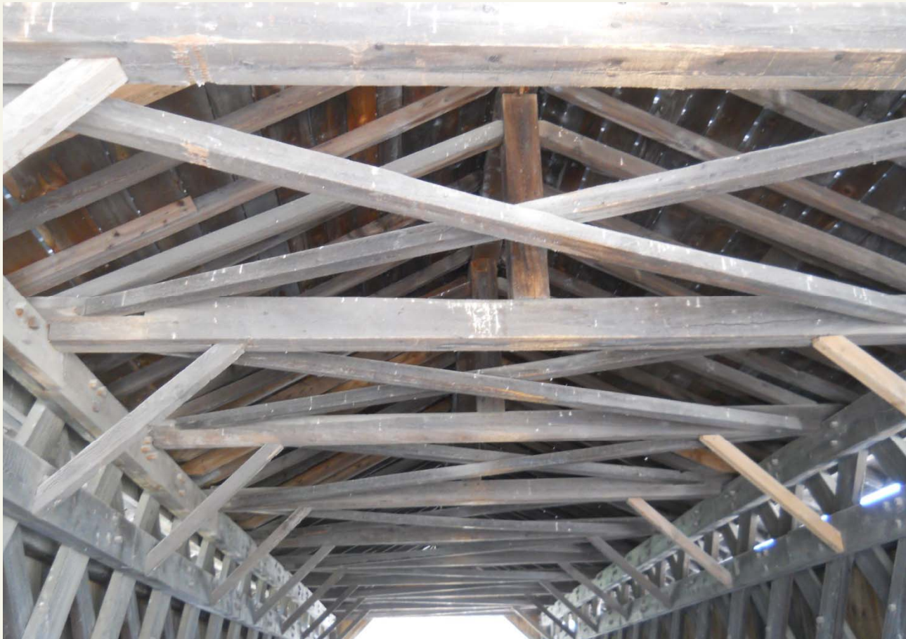
Longley Covered Bridge (Built 1863) – Montgomery, VT
