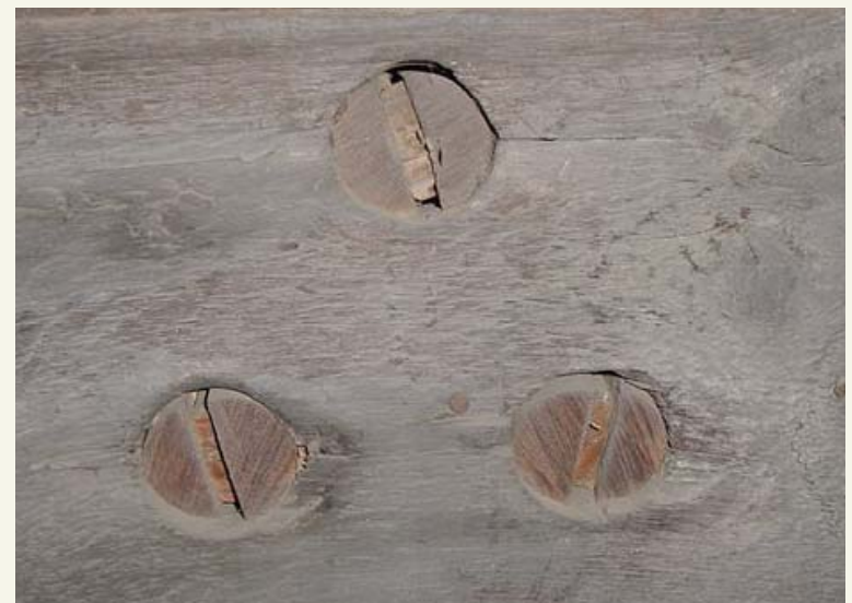
Trunnels with Wedges – Haverhill-Bath, NH Covered Bridge (Built 1827-1829)
