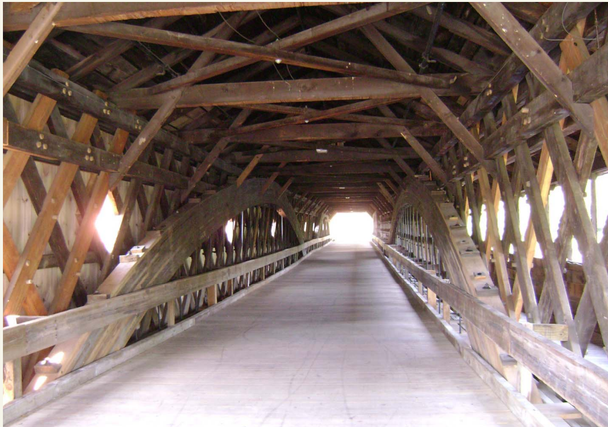
Haverhill-Bath, NH Covered Bridge (Built 1827-1829)
