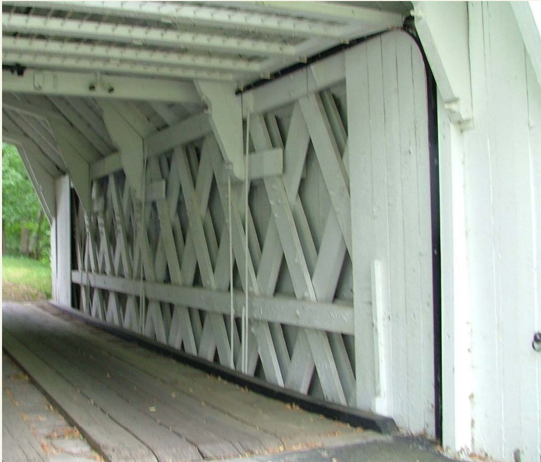
Cousineau Bridge over Brandy Creek at Valcourt (Built 1888) (61-66-02) Photo Courtesy Jack Schmidt – 6-30-11
