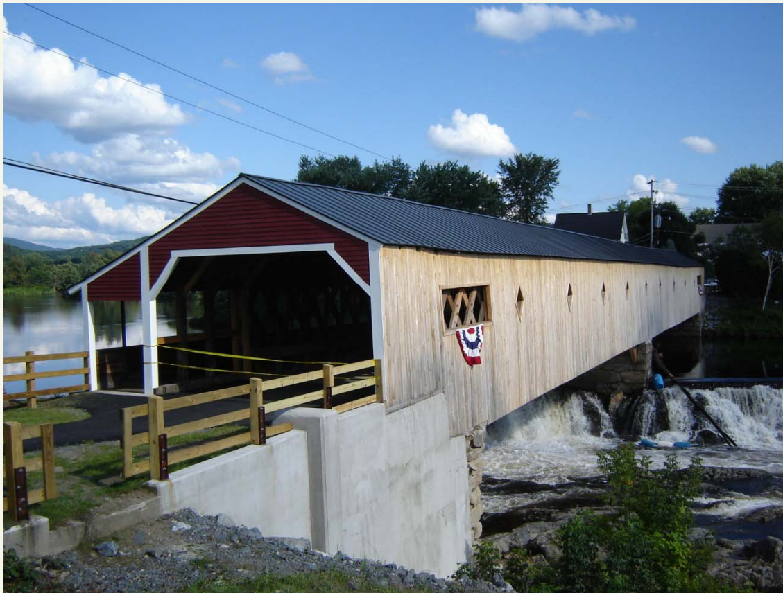
Haverhill-Bath, NH Covered Bridge (Built 1827-1829)
