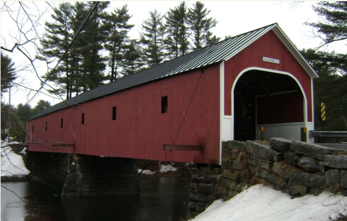
Cresson Covered Bridge (Built in 1859) – Swanzey, NH
