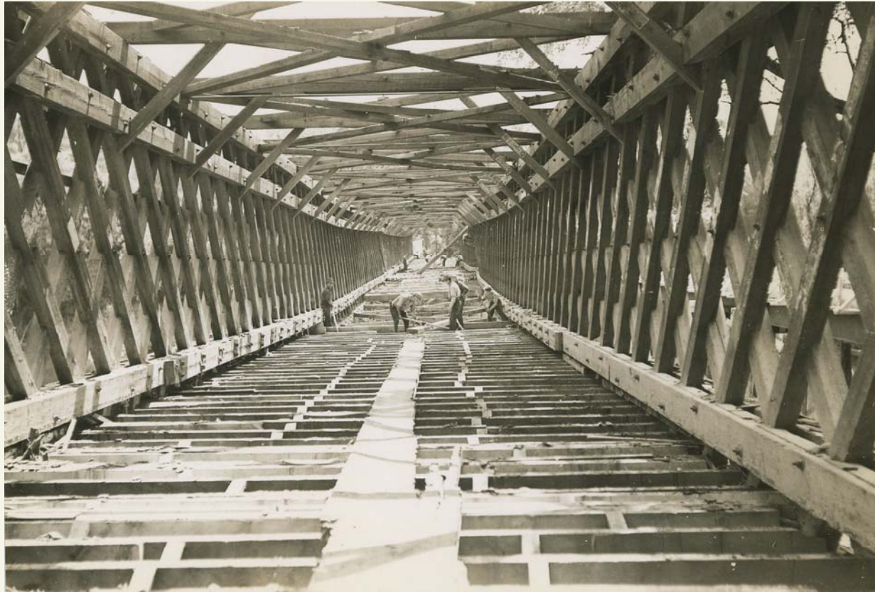
Orford-Fairlee Covered Bridge (1856-1936) – Photo Courtesy George Pease Collection, NSPCB
