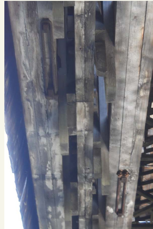
Fisher Bridge (Built 1908) – Wolcott, VT
