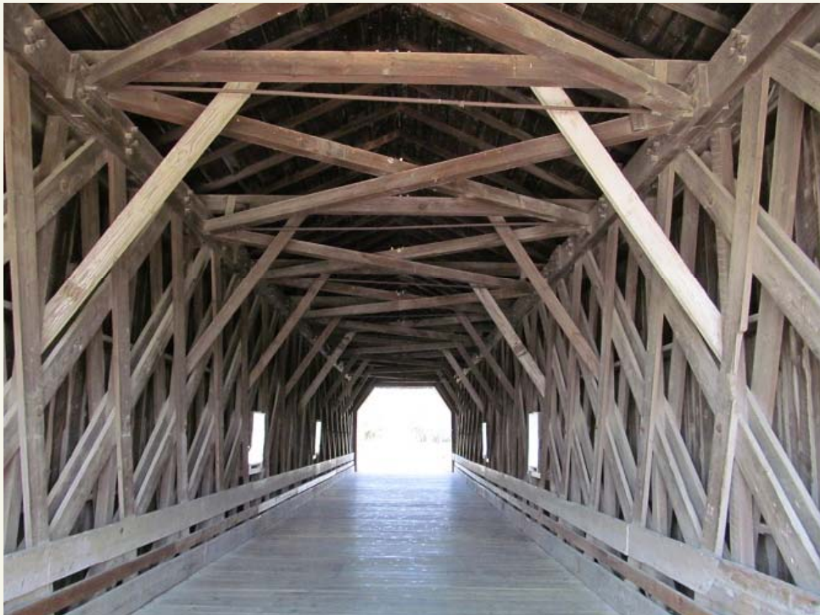
Zumbrota Covered Bridge (Built 1869) – MN
