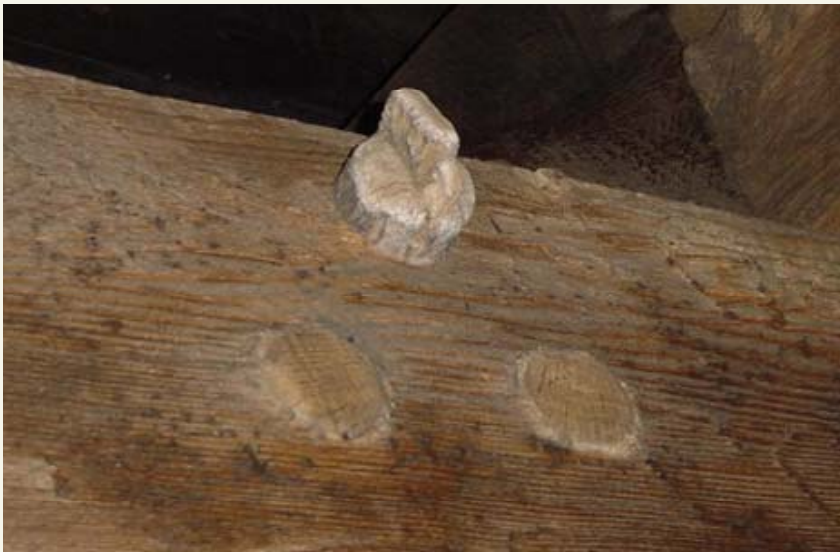
Trunnels with Wedges – Haverhill-Bath, NH Covered Bridge (Built 1827-1829)
