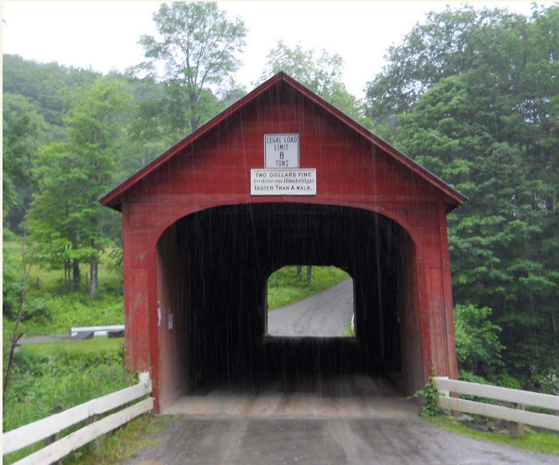
Green River Bridge (Built 1870) – Guilford, VT
