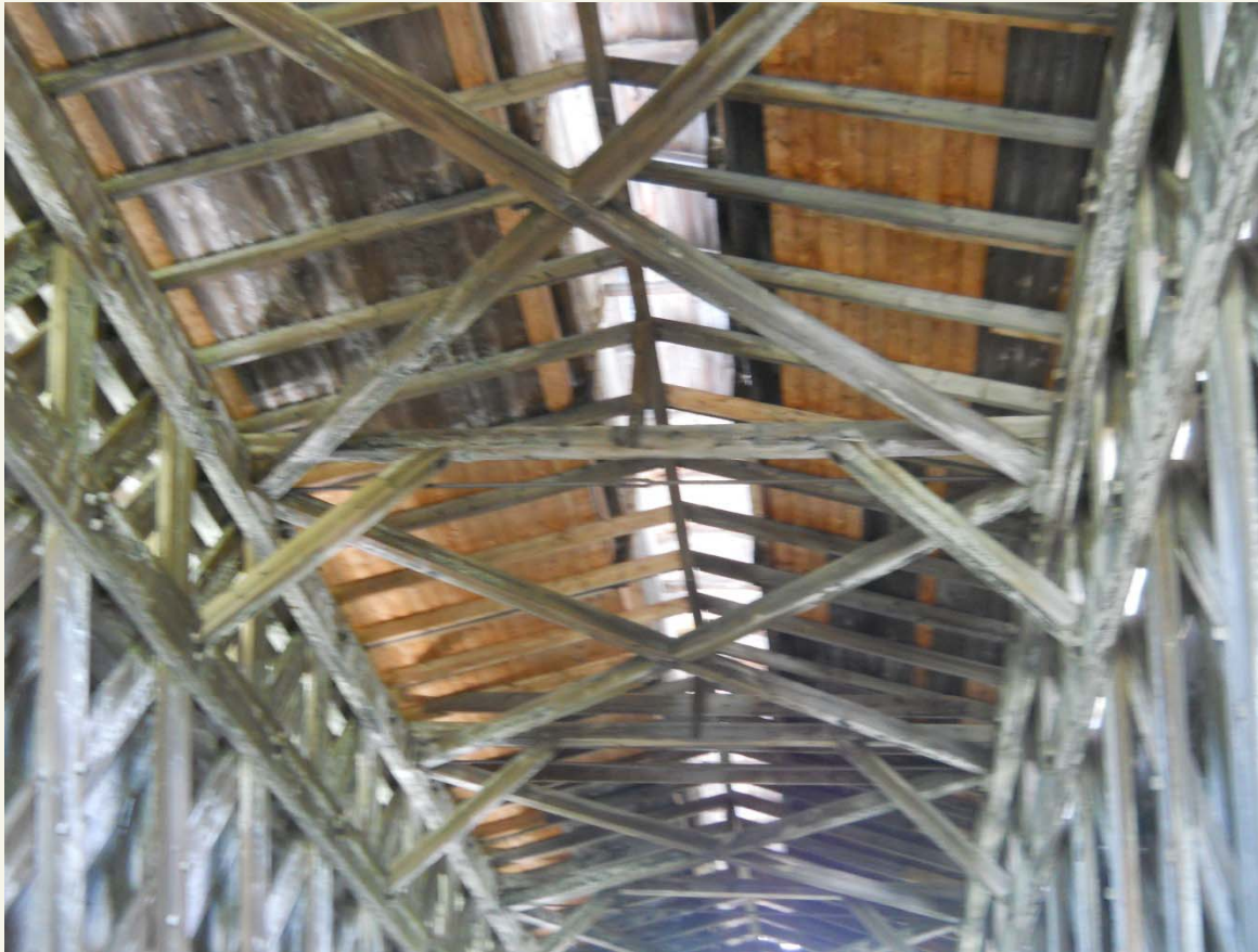
Fisher Covered Bridge (Built 1908) – Wolcott, VT
