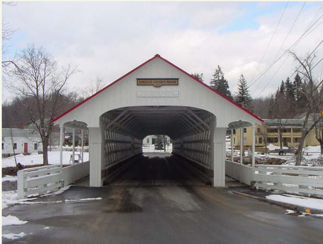
Ashuelot Covered Bridge (Built 1864) – Winchester, NH
