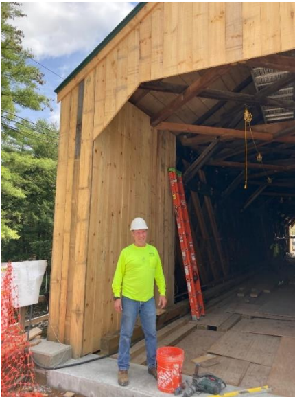
Pictured is Jim Ligon standing at east portal of the nearly finished Kingsley covered bridge. Photo by Beth Brown Limmer
