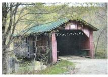
The Hutchins Covered Bridge was inspected and load rated to determine its current condition. Our rating assumes replacement of deteriorated bridge members. It was determined that at the inventory stress limit, the existing trusses have a live load capacity of approximately H7.8 (7.8 tons), the floor beams have a capacity of H4.2 (4.2 tons), and the deck has a capacity of H7.2 (7.2 tons).
