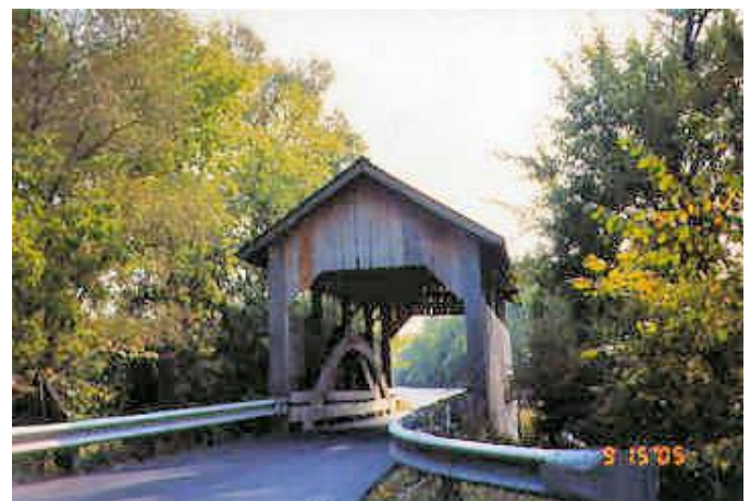
Lakeshore Bridge, photo by Tom Keating, September 2005
