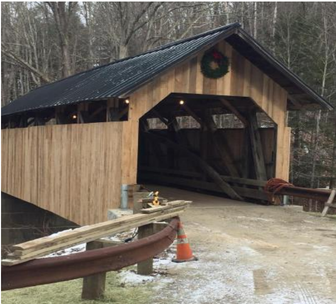
Seguin Bridge, photo courtesy of VTrans
