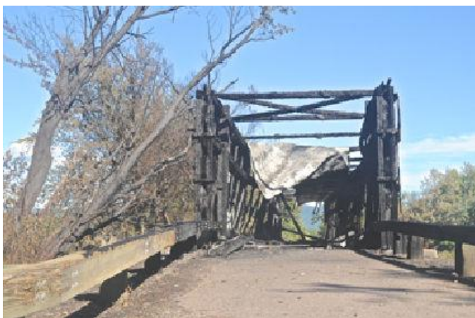
Salisbury Station Bridge photo by Ed and Irene Barna, September 11, 2016
