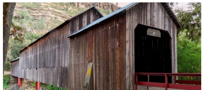
Honey Run Covered Bridge
