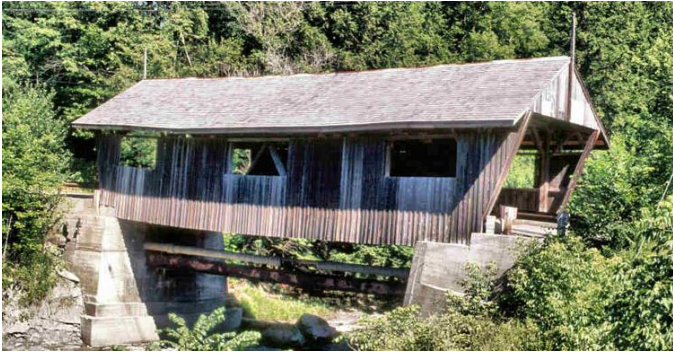
Power House Bridge by Joe Nelson
