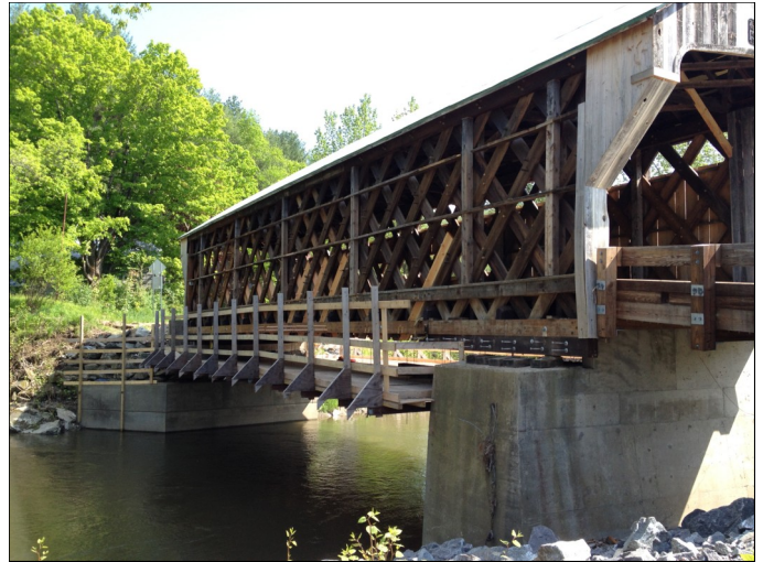
Worrall Repairs May 2012 - photo by Adrienne Hitchcock
