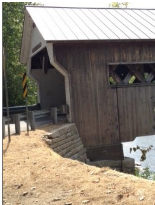
Dummerston Bridge east portal approach and wingwall 8/12/12 A. Hitchcock
