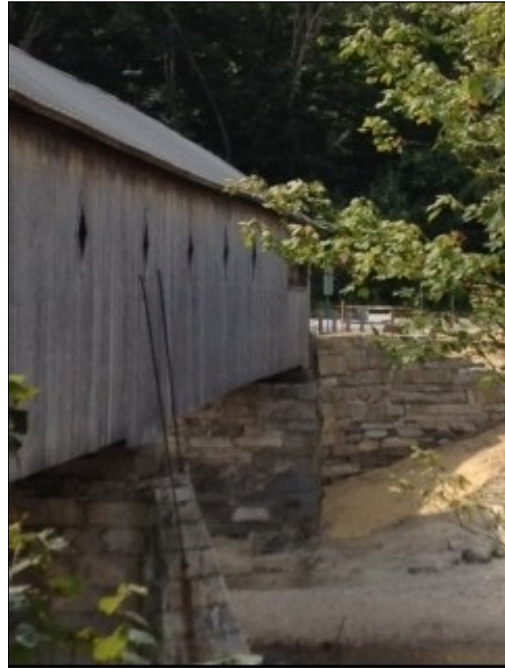
Dummerston Bridge west portal and wingwall 8/12/12 by A. Hitchcock
