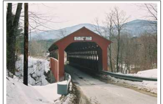
East Arlington Bridge (WGN 45-02-05) © 2003 Richard St Peter
