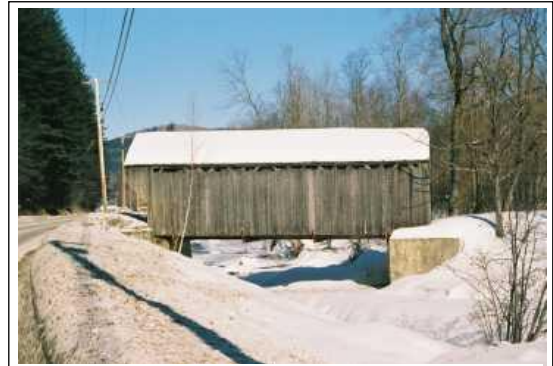
Giorgetti Bridge, Pittsfield, Vt. (45-11-B2) 1978 stringer © 2003 Richard St Peter
