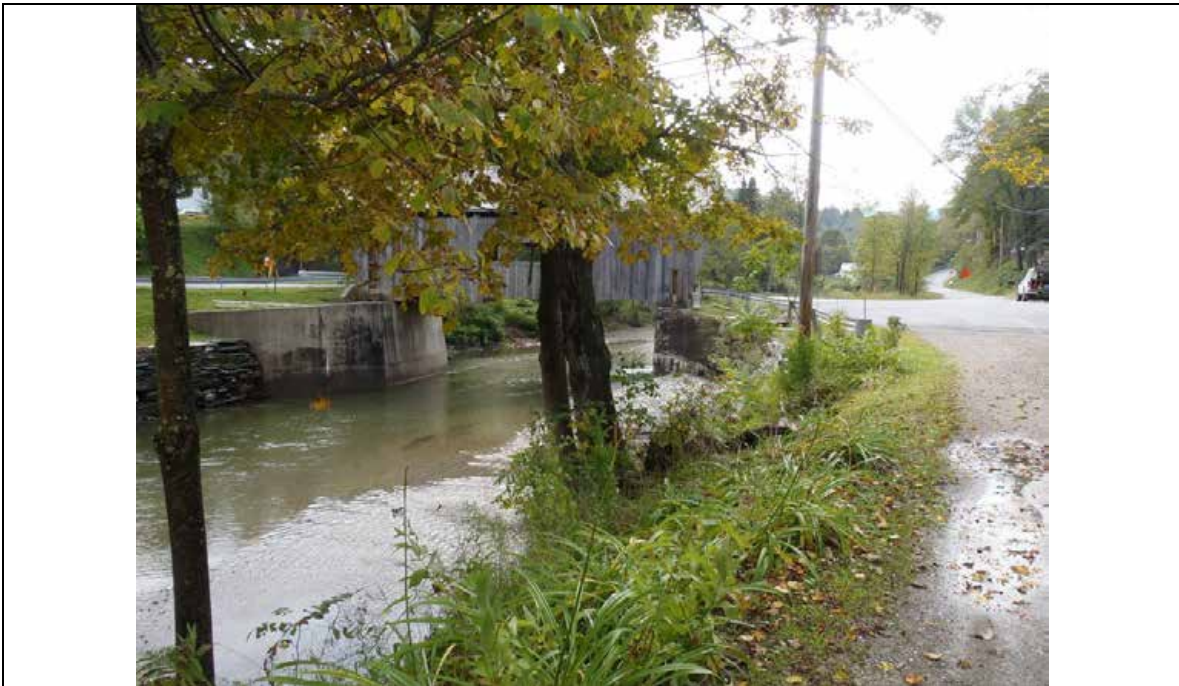
Mad River - Covered Bridge looking upstream
