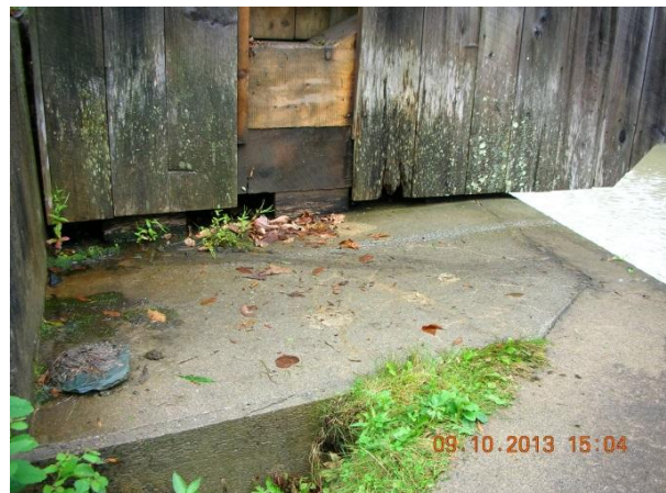
East Abutment Bearing Seat Subsidence
