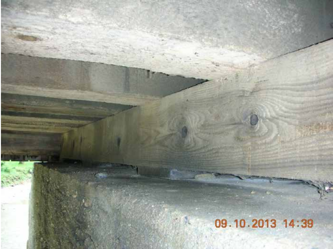
Photograph 5 - Ends of Stringers and Stringer Bearing Beam
