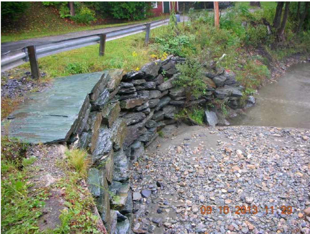
Photograph 9 - Retaining Wall (Downstream Side, West Bank)
