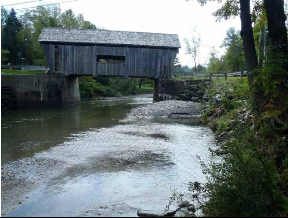
Mad River - Covered Bridge looking upstream
