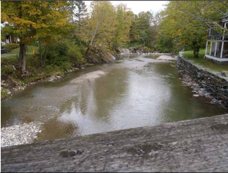
Mad River - Covered Bridge looking down toward the dam.
