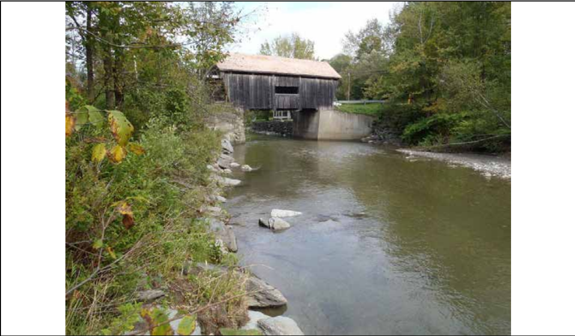
Mad River - Covered Bridge looking downstream. (Looking north).
