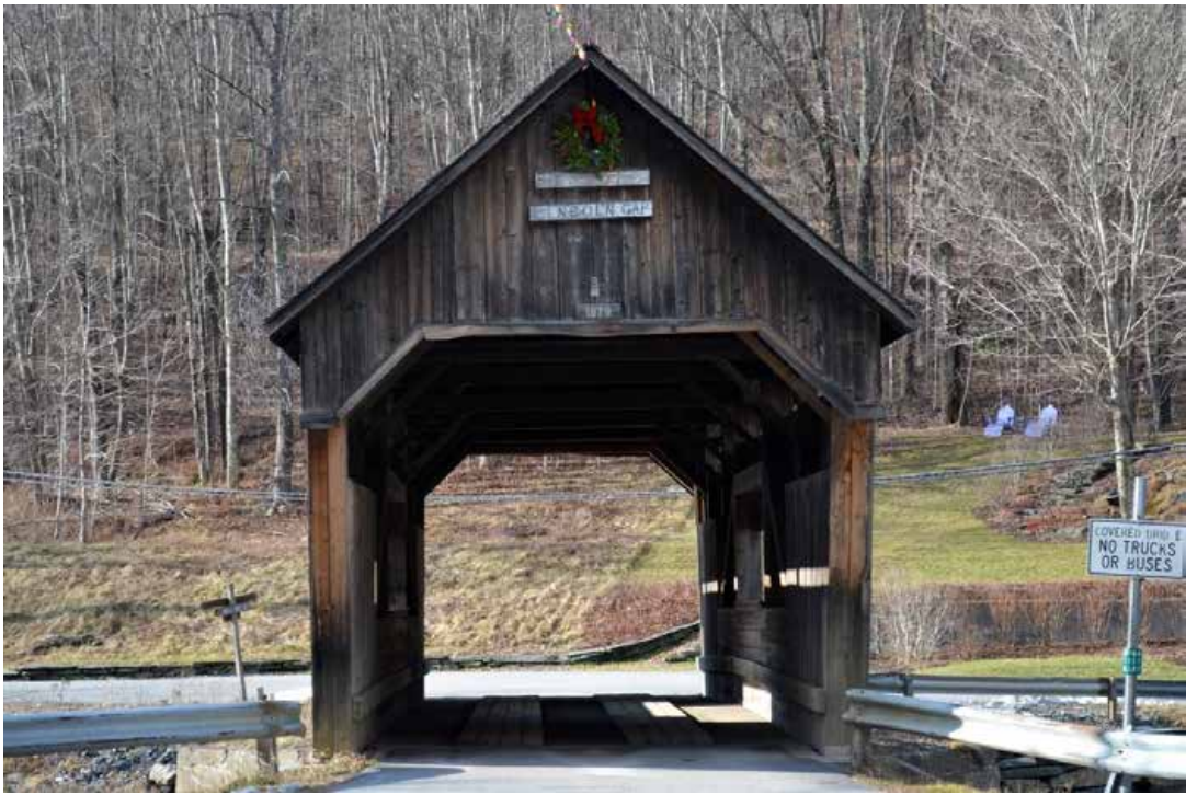
Photograph 7 - Portal at East End
